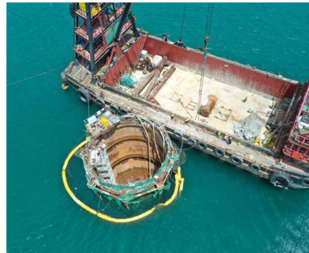
Retrieval of tunnel boring machine at outfall cofferdam
