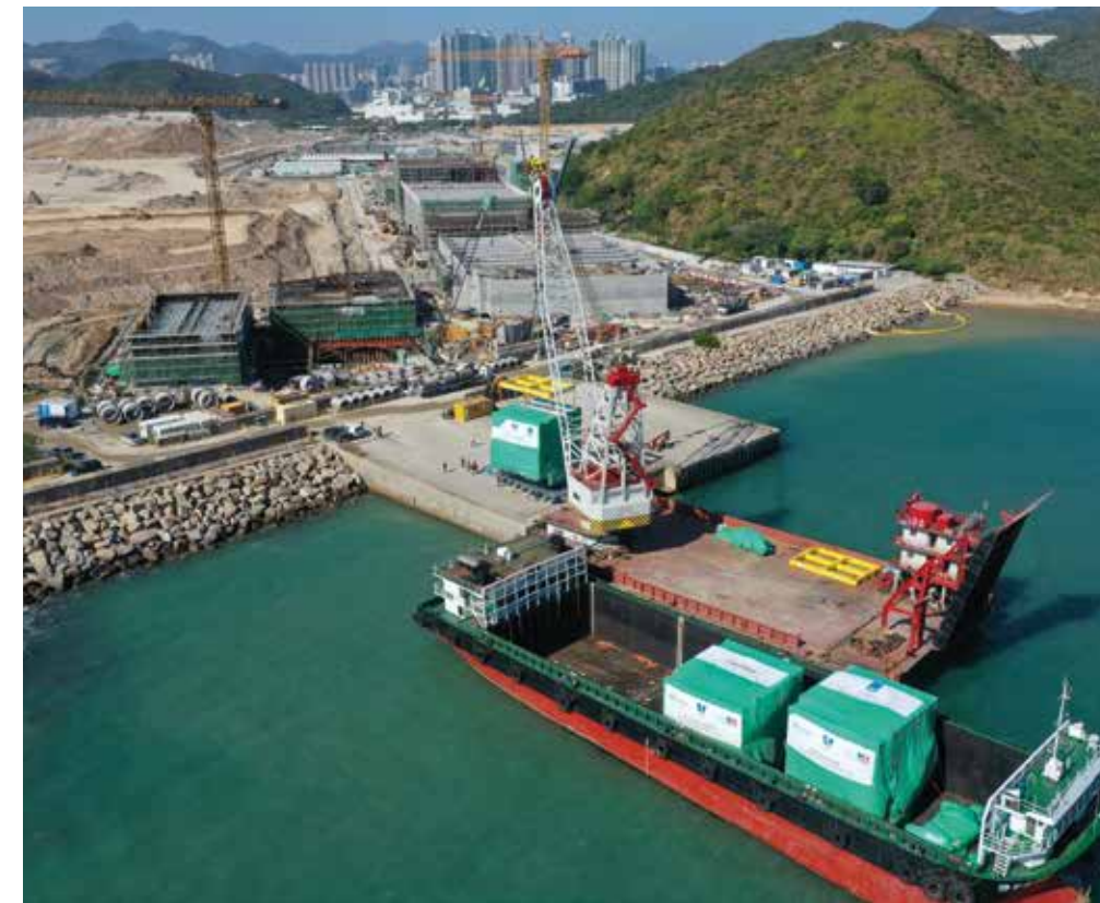
Delivery and installation of reverse osmosis modular skids
