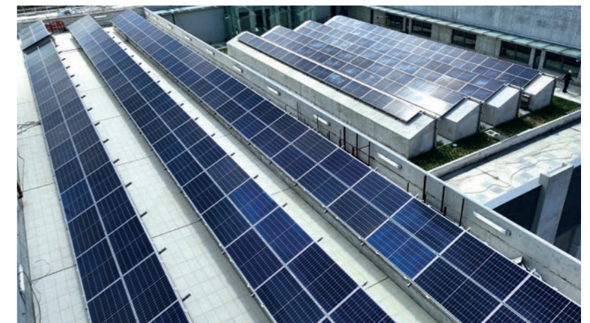
Above: photovoltaic (PV) panels will help to power the desalination plant. Left: soft landscaping helps to mitigate the 'heat island' effect of the new buildings as well as providing aesthetic appeal
